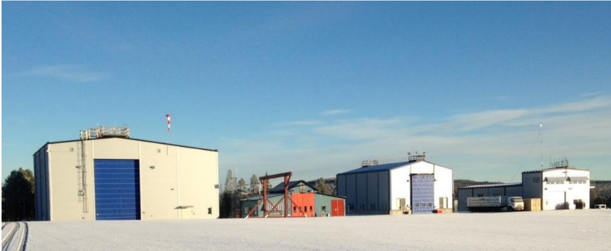
Figure 19 - From left to right: the Dome, the Chapel, Cathedral and Basilica preparation & assembly buildings
