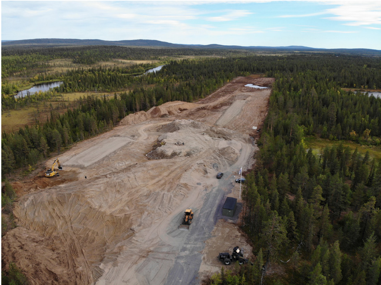
Fig. 7 - Status of LC-3 site development (as of Sep 2020)
