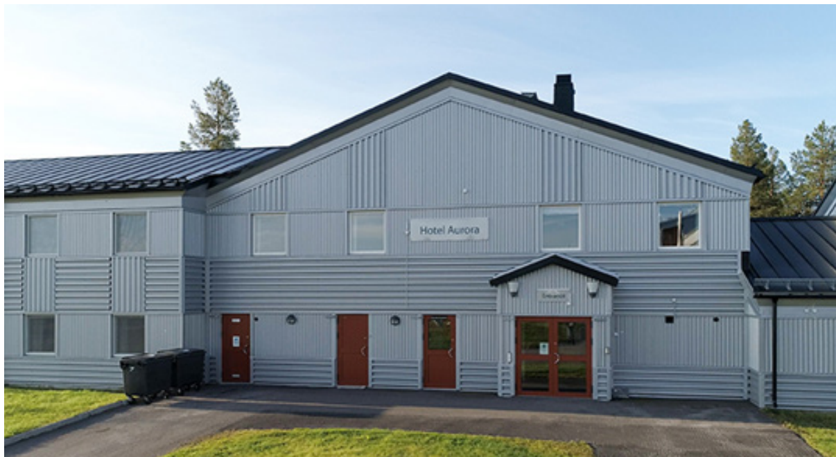
Fig. 21 - Main entrance to Hotel Aurora
