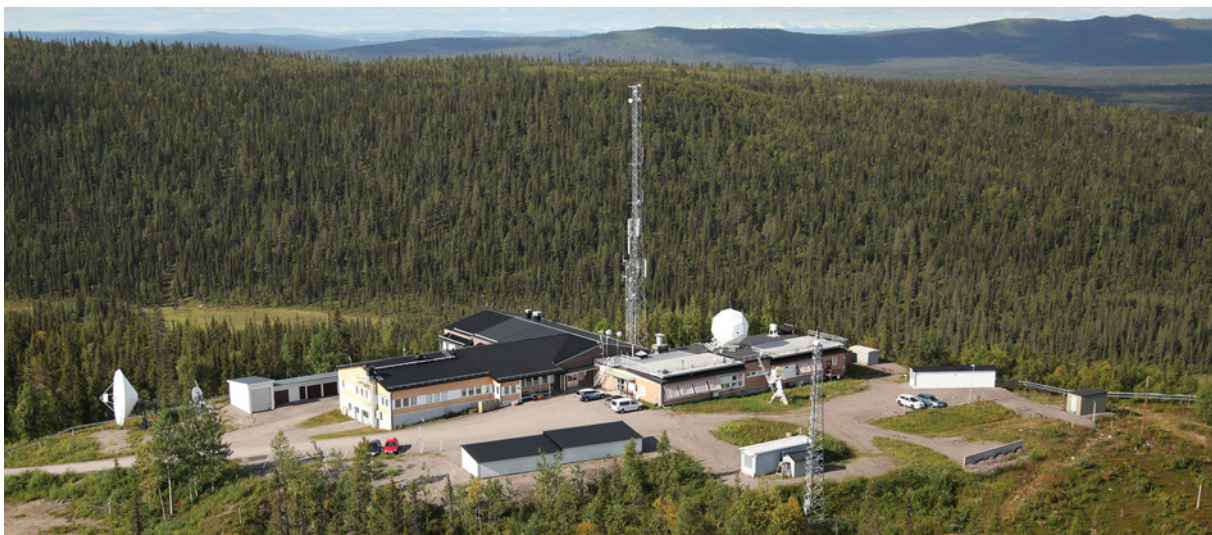
Fig. 8 - Satellite Station on Radar Hill
